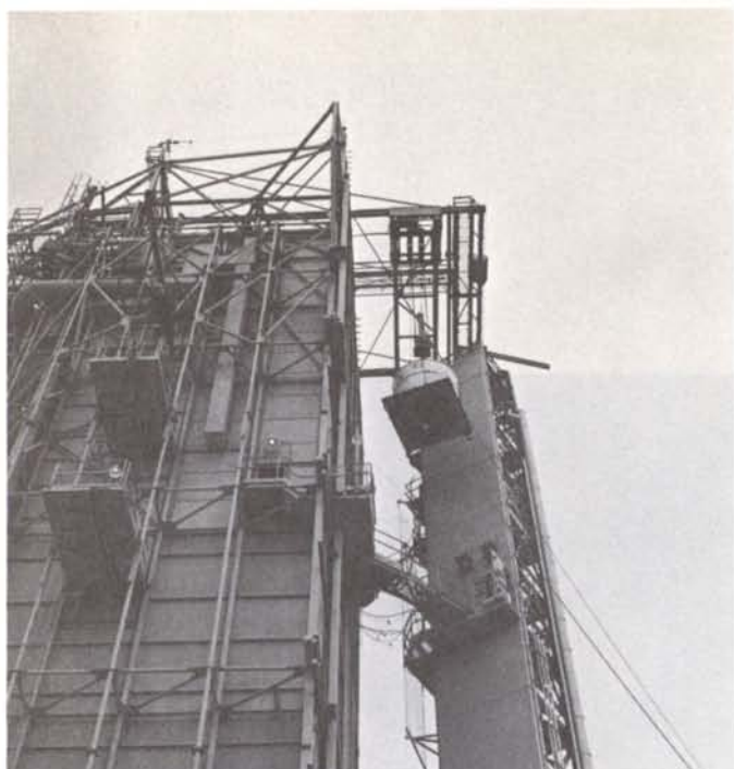
Hoisting the satellite in container to gantry Level Six
